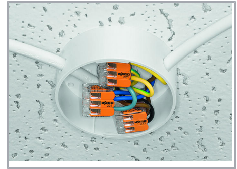
Lighting distribution in ceiling canopy
