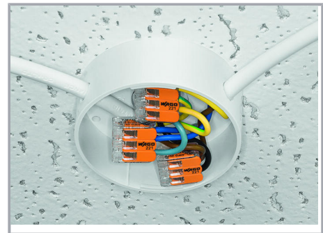
Lighting distribution in ceiling canopy
