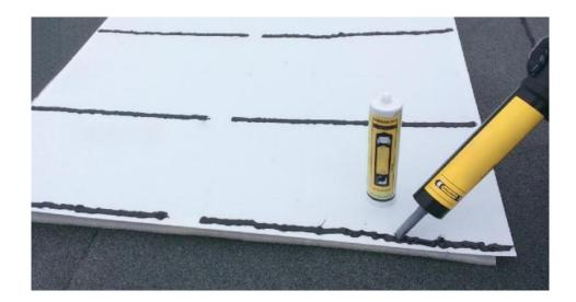
The adhesive lines can be as close to each other as required (the number of lines depends on the strength your chosen adhesive), but a minimum gap of at least 70 mm between lines is recommended. In general, for most plastic / fibreglass / metal surfaces and a good quality adhesive, a gap of 100 - 150 mm between parallel adhesive beads would form a strong bond.
